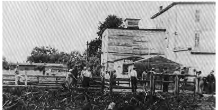
Flood in 1935, Cambridge Mill.
